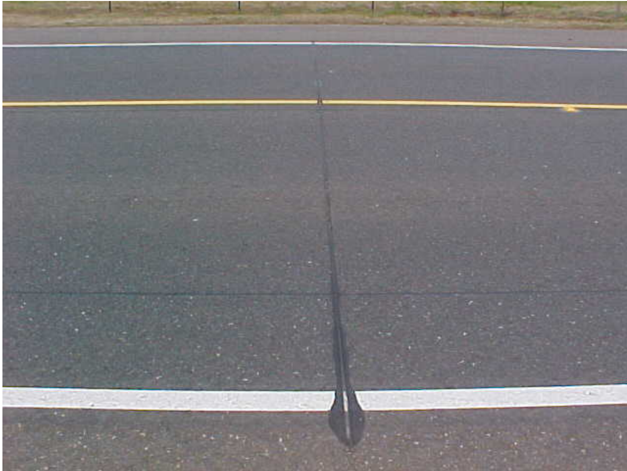
Completed Overlay With Sawed and Sealed Joints
