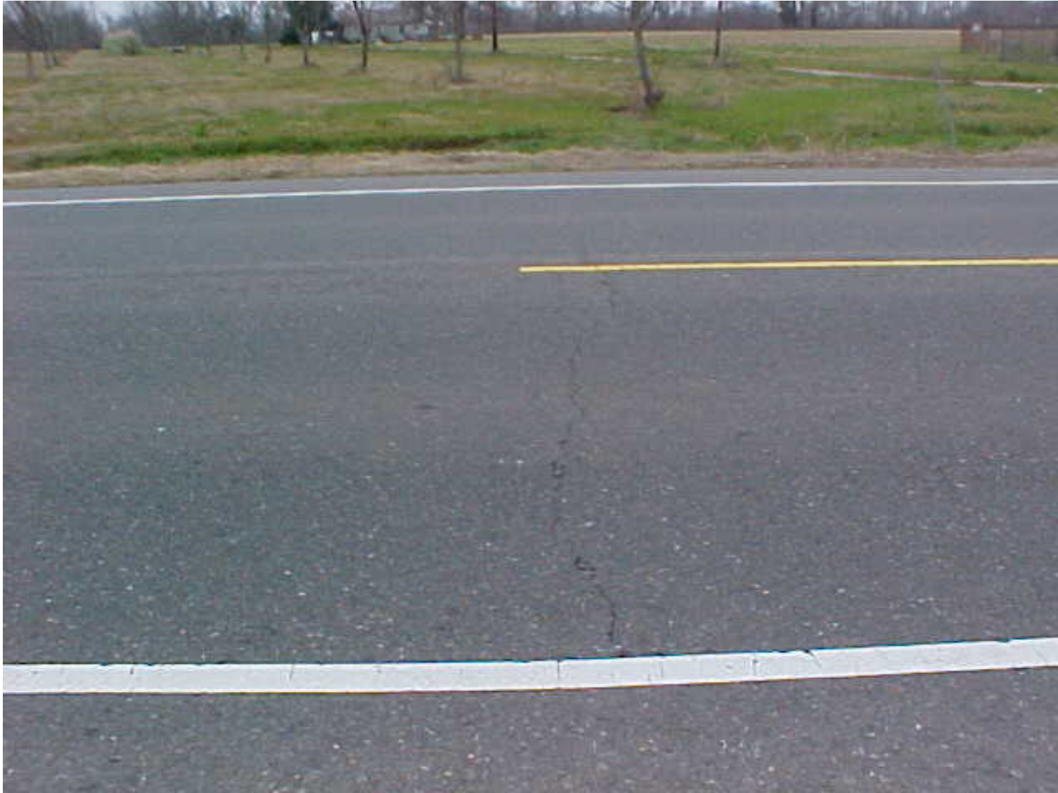
Completed Ultra-Thin Overlay
