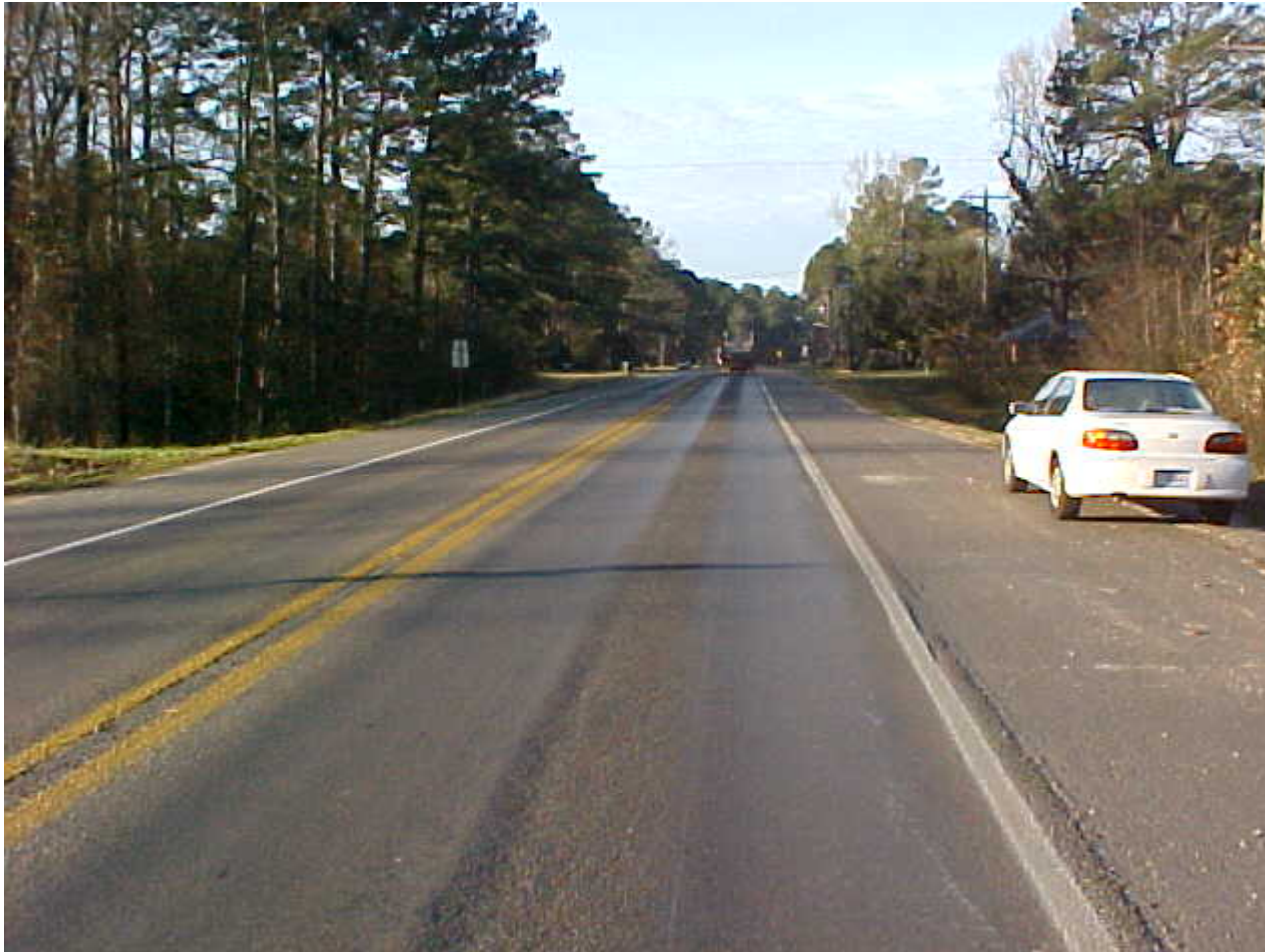
Completed AST Project (Polishing In Wheel Paths)
